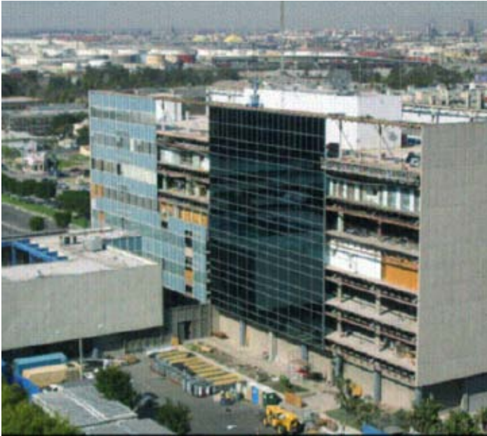
Long Beach Public Safety Building during remodeling
