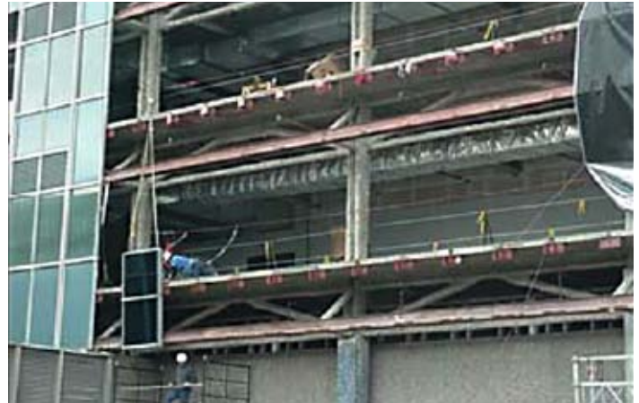
Curtain wall replacement.
