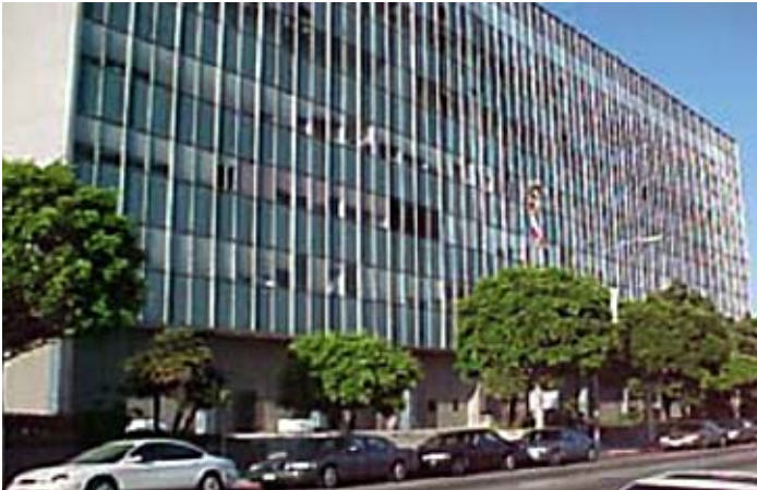
Before the renovation.
